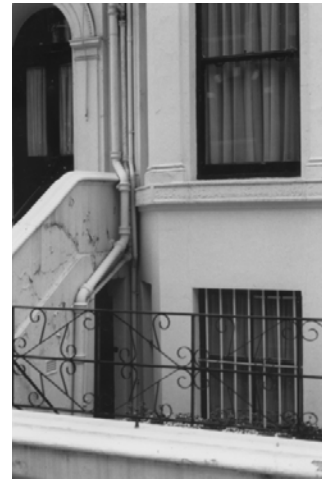
16. Window of Jones's room, 12 Sheffield Terrace
